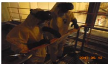
5. Set up the blockade line for the Radiation Leakage Area
